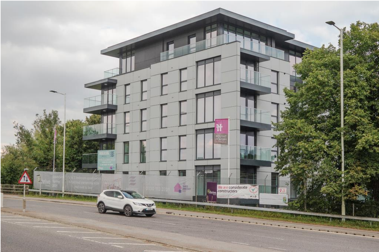
Rent to buy housing at Two Waters Road, Hemel Hempstead
