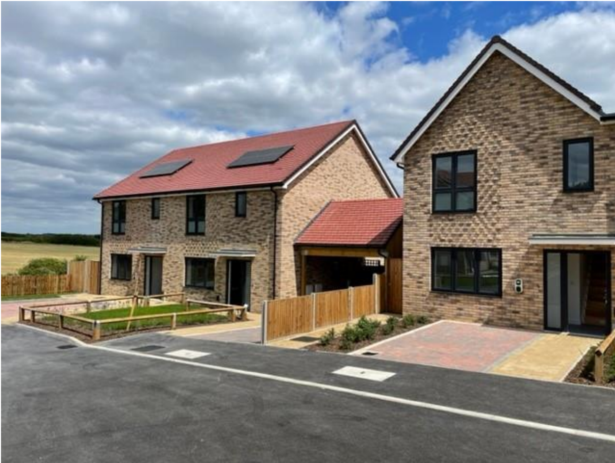
Recently completed Council homes on Coniston Road, Kings Langley
