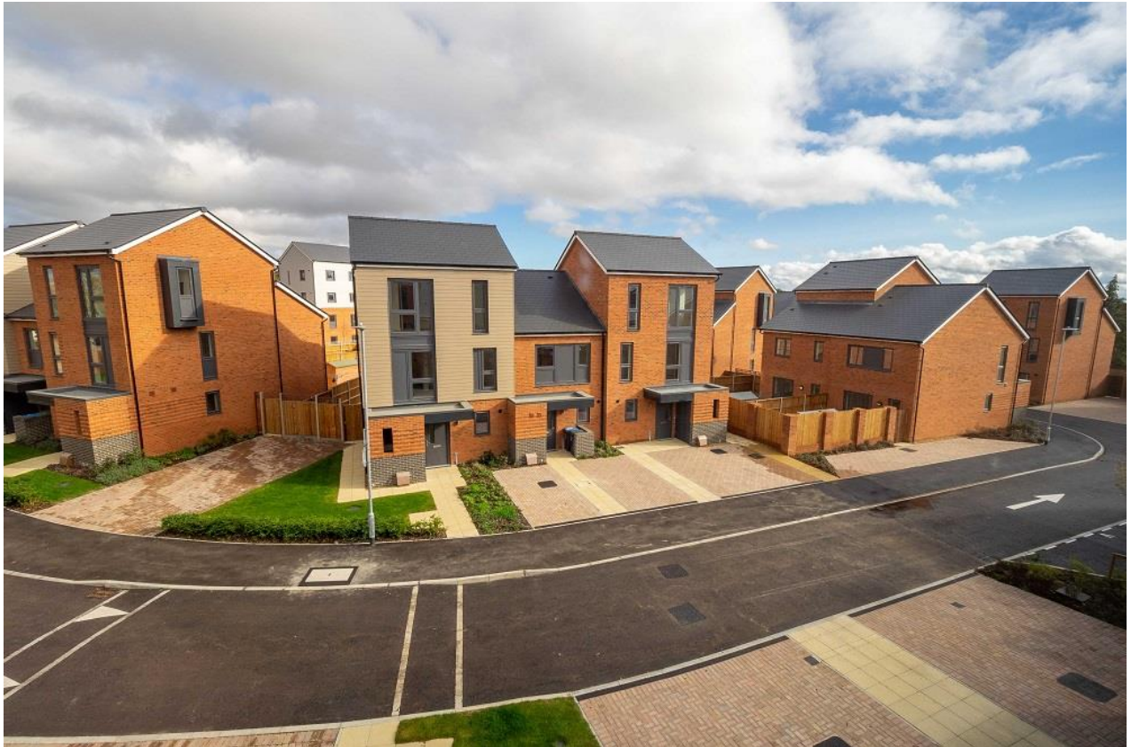
Recently completed Council Homes at School End Crescent and Old School House, Hemel Hempstead
