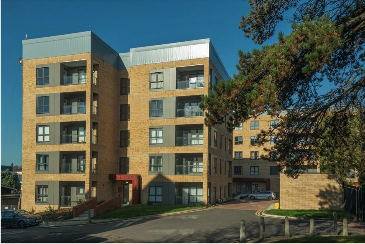
Affordable rented housing at Wood Lane, Paradise, Hemel Hempstead (Hightown Housing Association)
